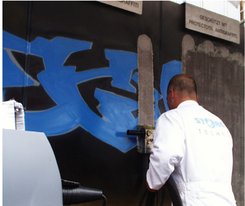
Cleaning of a wall with graffiti art
