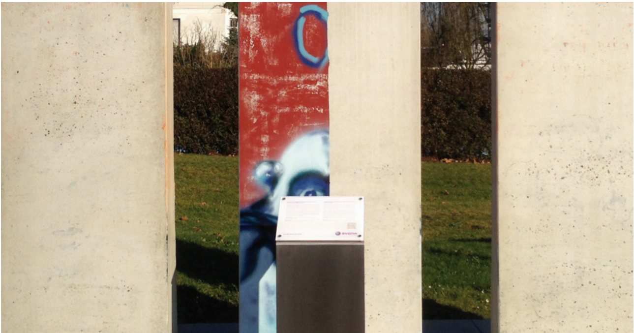
Concrete wall after removal of graffiti
