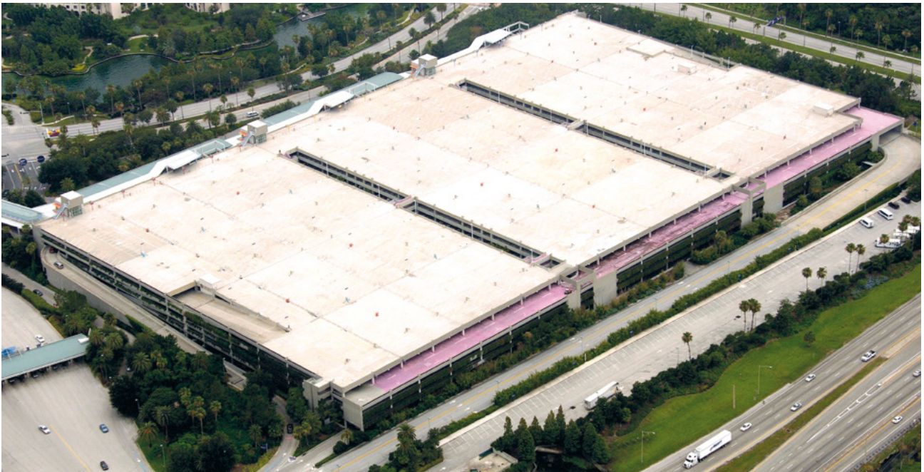
The parking areas of Universal Studios in Orlando, Florida, USA have been protected against corrosion by Protectosil® CIT
