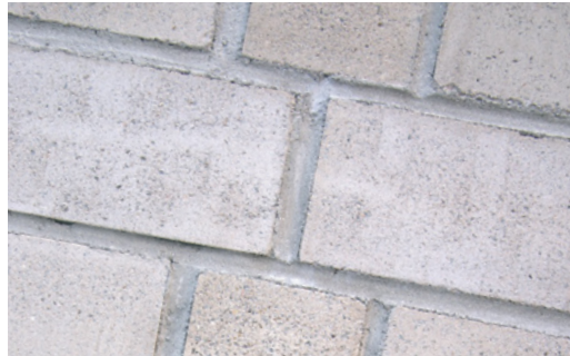
Treated with Protectosil® SC CONCENTRATE (without cleaning)
