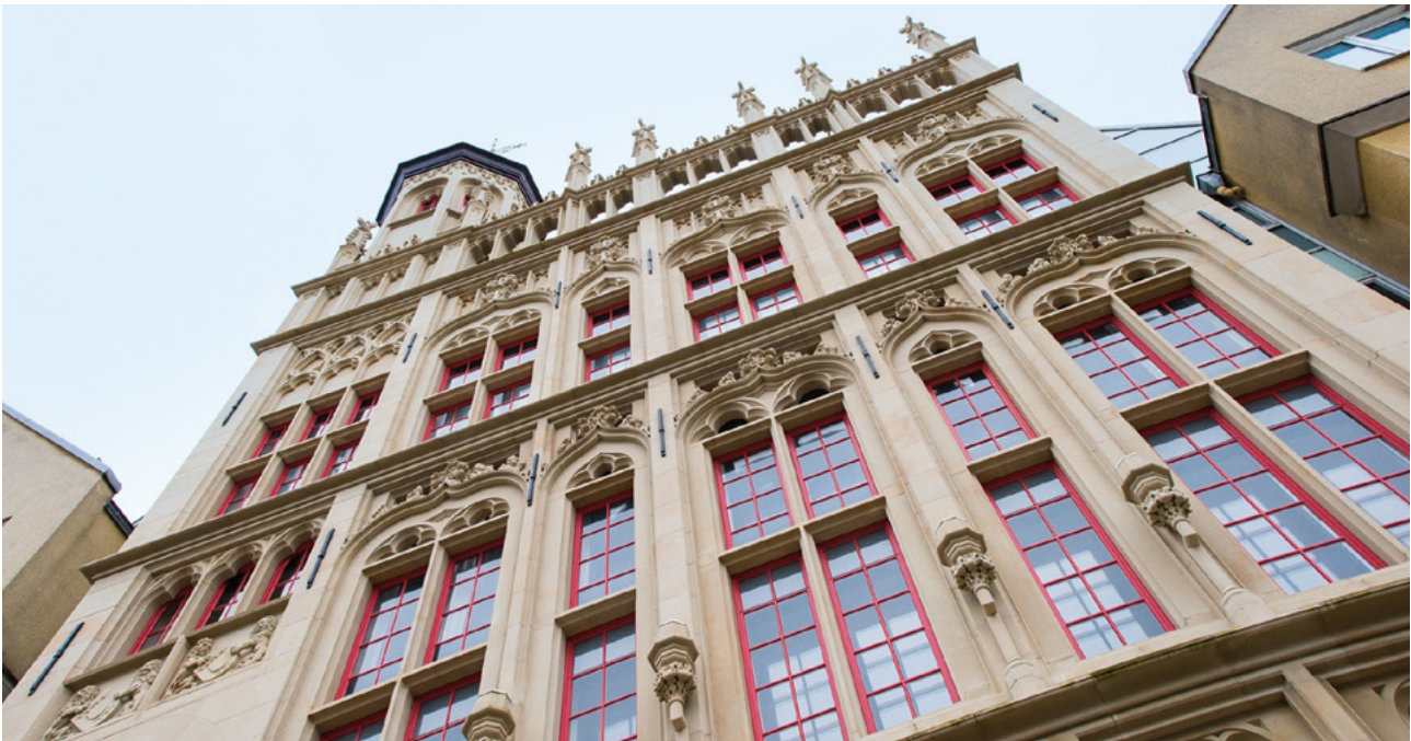
Protectosil® shields the facade of the City Hall in Wesel, Germany
