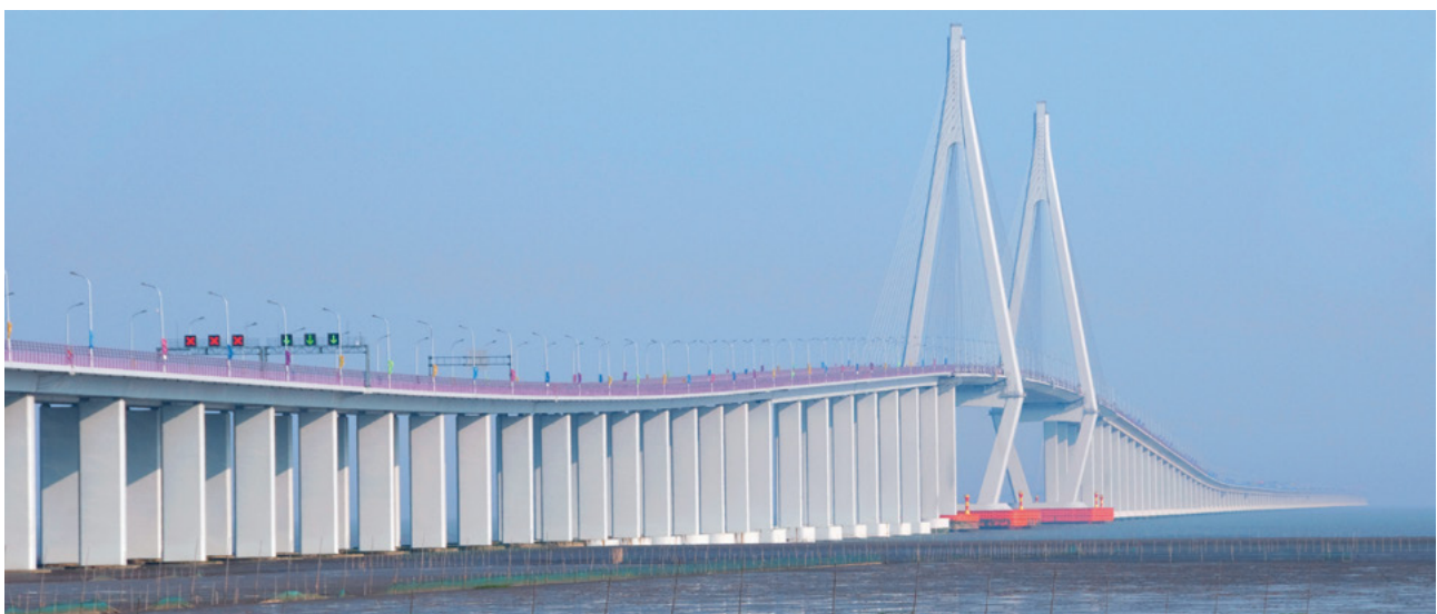
The 7,000 piers of the Hangzhou Bay Bridge in China are anchored in the seabed. Protectosil® CIT protects them against penetration of water and chemicals
